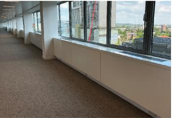
Even this tower block required bespoke components. The refurbishment of five floors of these offices required over 800m of fan coil casings. The structure itself creating identical bays with two active sections and a central make up section concealing the pipework. Skirting level cable trunking providing power without compromising the clean design. Bespoke end caps tied the deep casing back to the central services block while also covering the entry point of the large bore pipe work.
