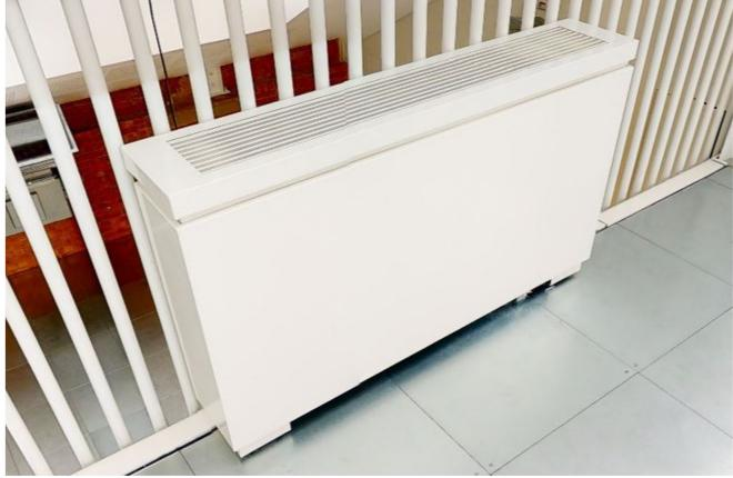
In this conversion of a former industrial warehouse. The fan coil units were situated along the balustrade either side of the mezzanine level, as well as around the exterior and stair cases. With an open view of the rear of the unit the design required a fully enclosed casing for the floor mounted FCU and the offset opening below the grille allowed for a shorter unit, maximising floor space.
